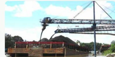
Coal loading w/ conveyor at load port/jetty
